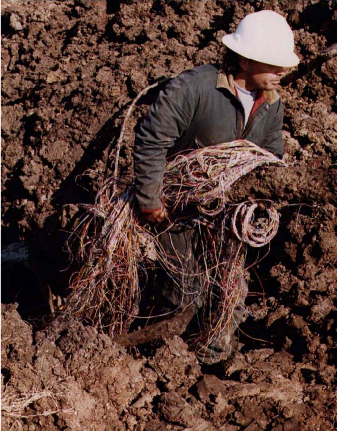
A Phone Company Worker responds to a severed 900 Pair cable
